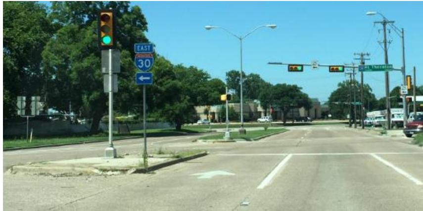
It is recommended for the City of Dallas to add signs for northbound and southbound left turns at IH 30 and Ferguson Road. A “Left-turn-yield-on-green” sign (MUTCD sign R10-12) at these intersections supplementing the left-turn signal heads is recommended.
